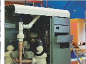
WATER PURIFICATION UNIT
