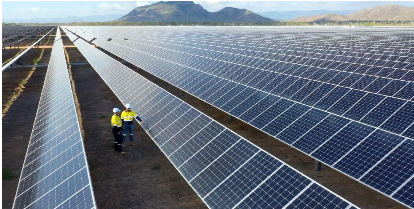
Ross River Solar Farm, QLD
