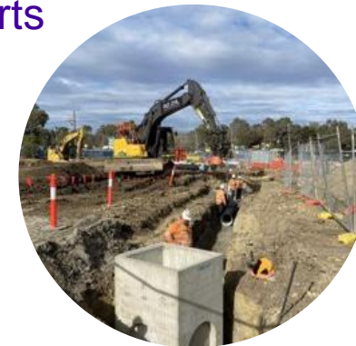
Trial of plastic pipe under pavement
